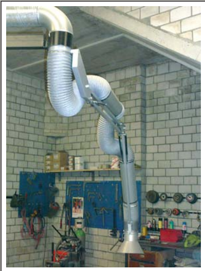
Boom arm with an extraction arm 160ø with pipes, external rods and hydraulic dampers for easy handling.
