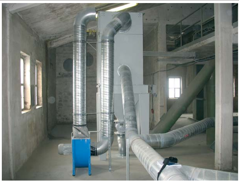
Atex-cartridge filter – central system with a capacity of 2000 m³/h for extraction in storage silos with worm gear discharge for medium feedback, including expansion flap.
