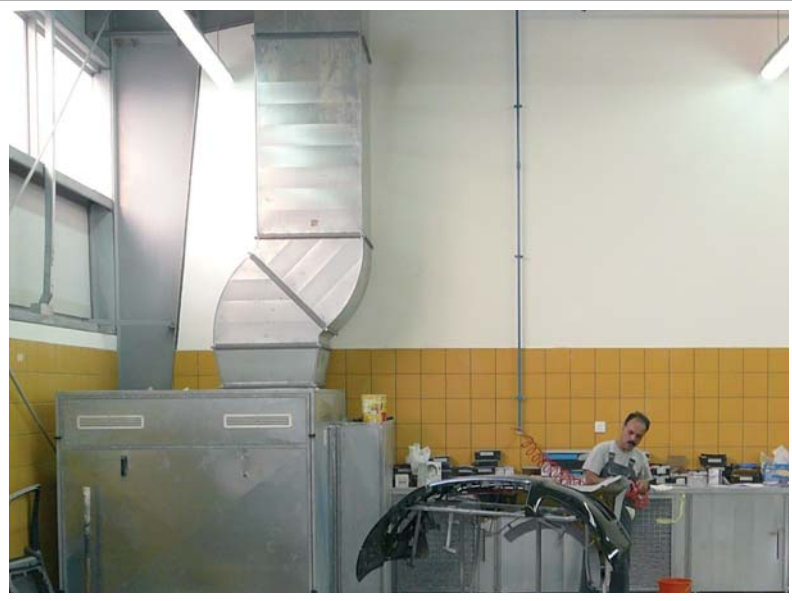
Primer surfacer/filler extraction in a varnishing preparatory hall.
