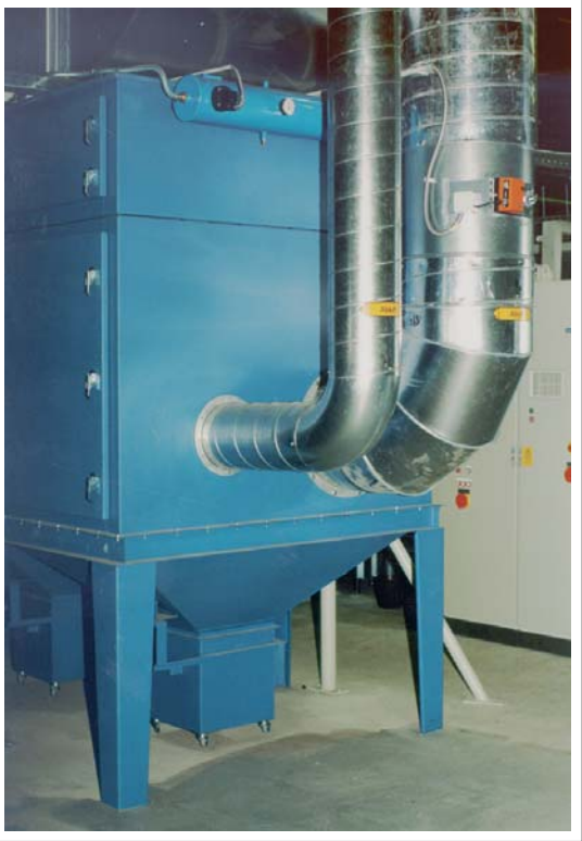
Cartridge filter – central system with a capacity of 12000 m³/h for welding and sharpening/grinding workplaces in train works.
